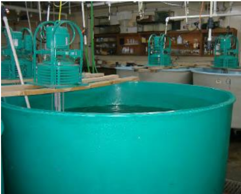
3000-liter broodstock holding tanks with chillers
