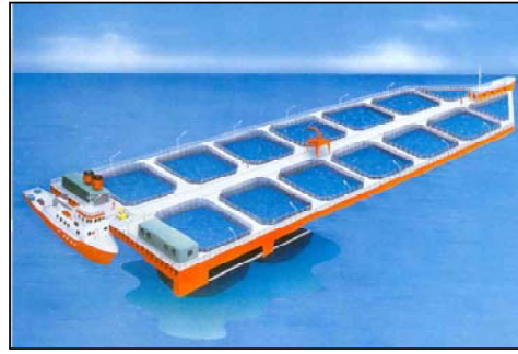
2. Viking Sea Going Farm circa 1988. Relied on strength to withstand ocean forces and failed.
