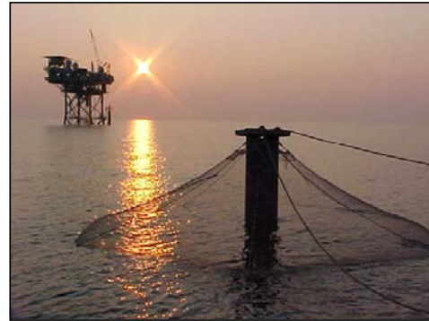
8. SeaStation single spar submersible cage, circa 1992. Fixed volume, tensioned rigging lines to support net, now in service in several countries
