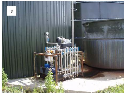
Figure 5.4 Meikle Laught on-farm biodigester a) 200m 3 digester tank, plant cabin and conditioning tank b) raw slurry in conditioning tank c) digestate d) plant in cabin, showing control panel, gas boiler and heat exchangers e) digestate storage tank, gas skids and gas store
