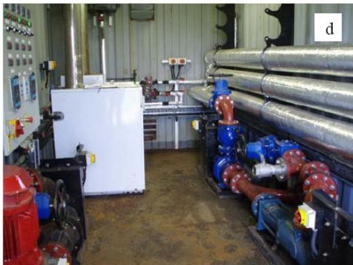
Figure 5.4 Meikle Laught on-farm biodigester a) 200m 3 digester tank, plant cabin and conditioning tank b) raw slurry in conditioning tank c) digestate d) plant in cabin, showing control panel, gas boiler and heat exchangers e) digestate storage tank, gas skids and gas store
