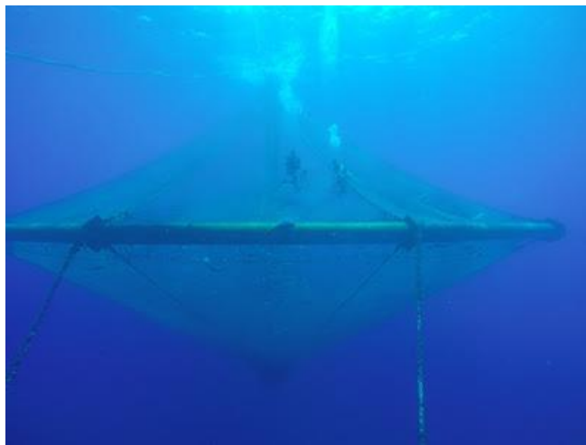
Figure 3 Submersible rigid cage (©InnovaSea Systems Inc)
